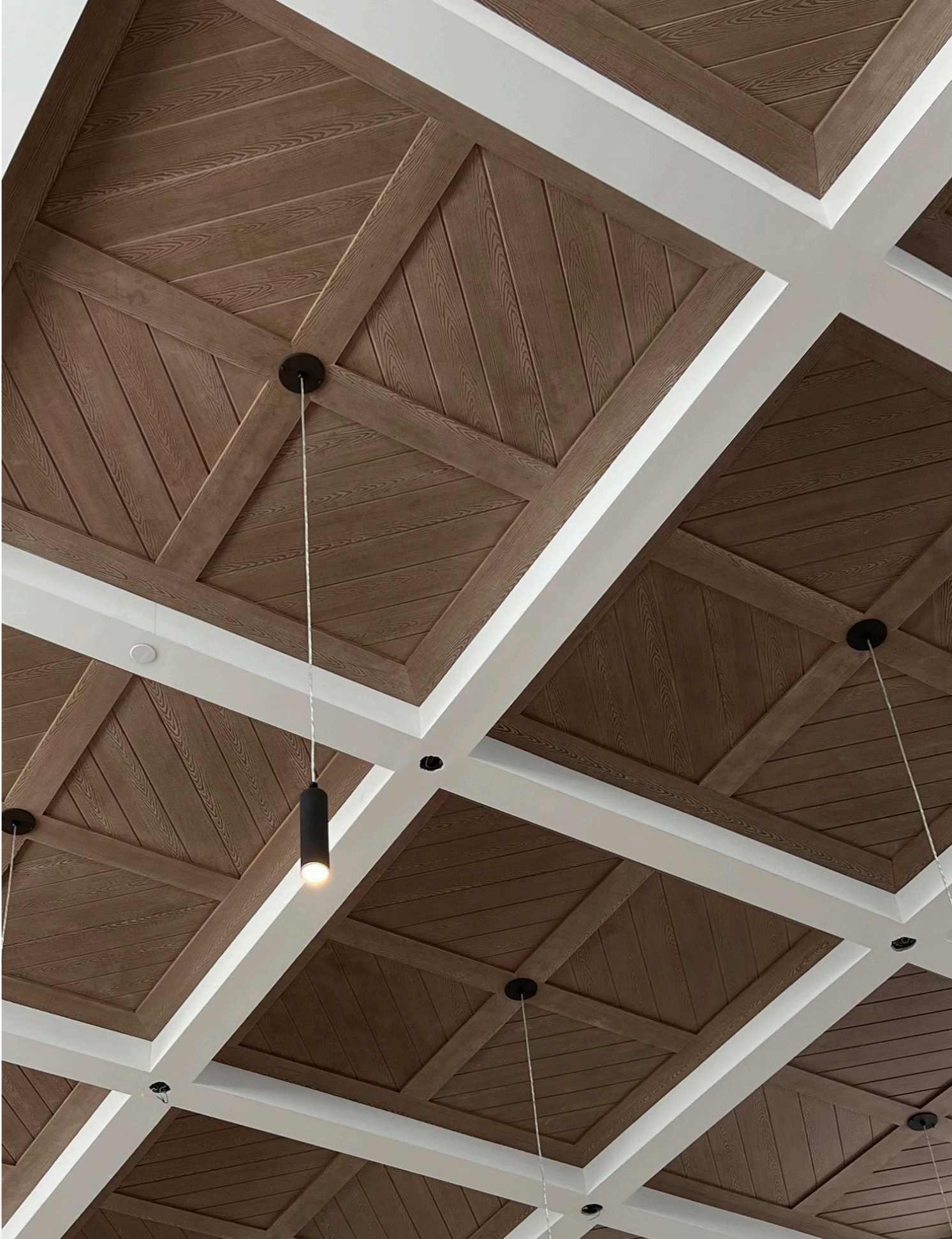
CEILING PANELS Miami, FL
